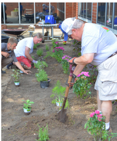
Volunteers and McGuire employees renovate the mental health patio garden with ultra-fine mulch, two flowerbeds and a raised bed. (Photo by Patrick Gordon)
